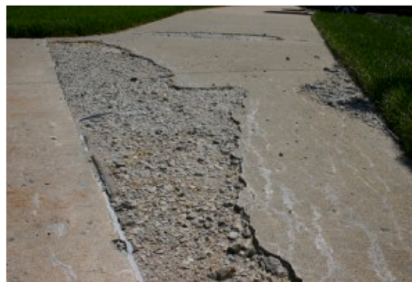
Fig. 12. Impact of freeze-thaw cycles on concrete.
